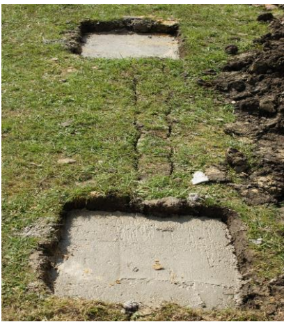
Typical Concrete Pad finish
