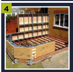
Attach brick skirt and modular wall to steel base and finish by fixing the bridging tiles in place.
