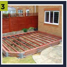
Attach the steel to the house wall, build and level the base using the adjustable legs.
