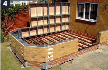
Attach brick skirt and modular wall to steel base and finish by fixing the bridging tiles in place.
