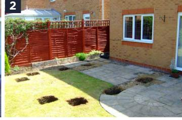
Install the concrete pads as per the pad plan supplied. Note the lack of mess and disruption!
