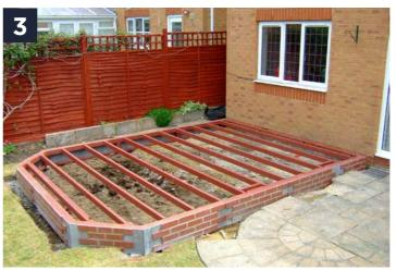
Attach the steel to the house wall, build and level the base using the adjustable legs.
